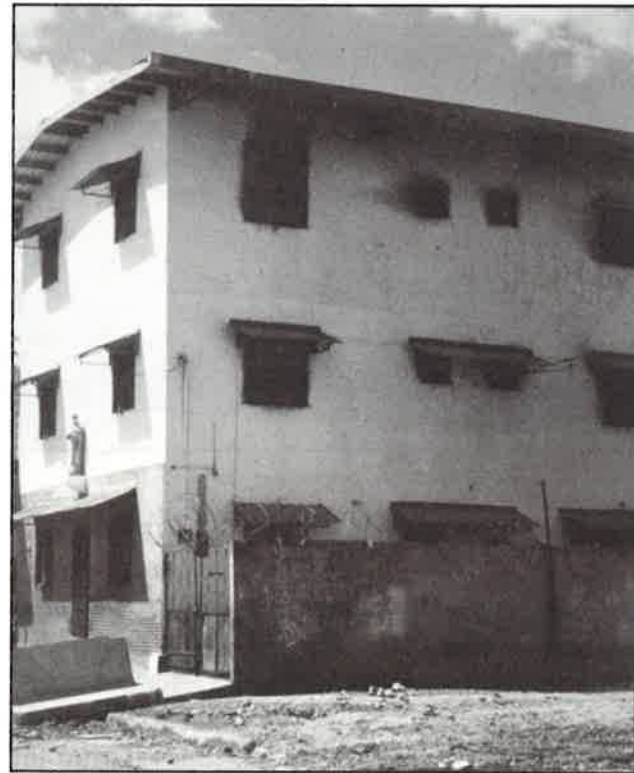
Masonry wall of Fatima Church where the fire was stopped.
