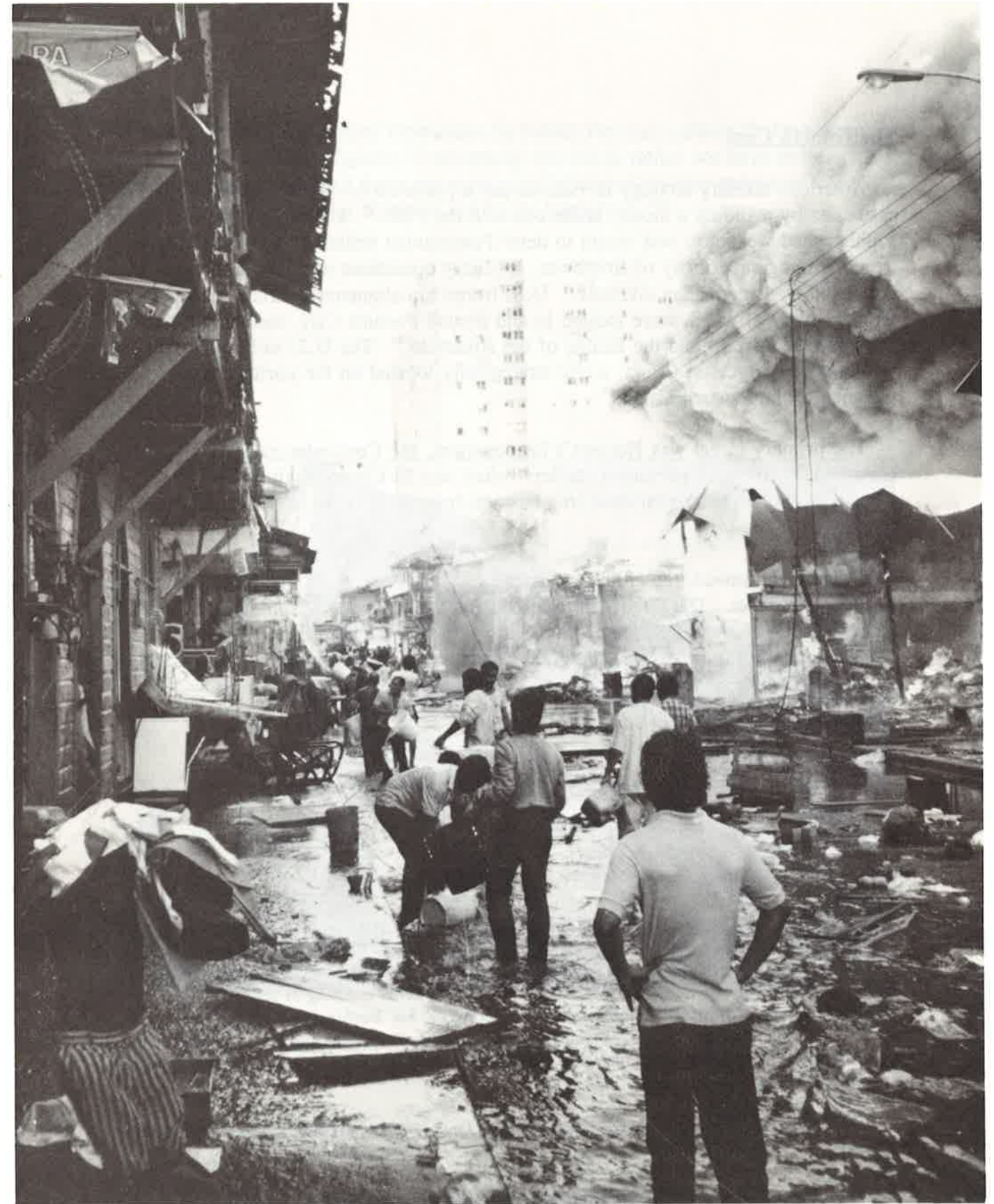
Chorrillo residents make desperate efforts to save buildings.
