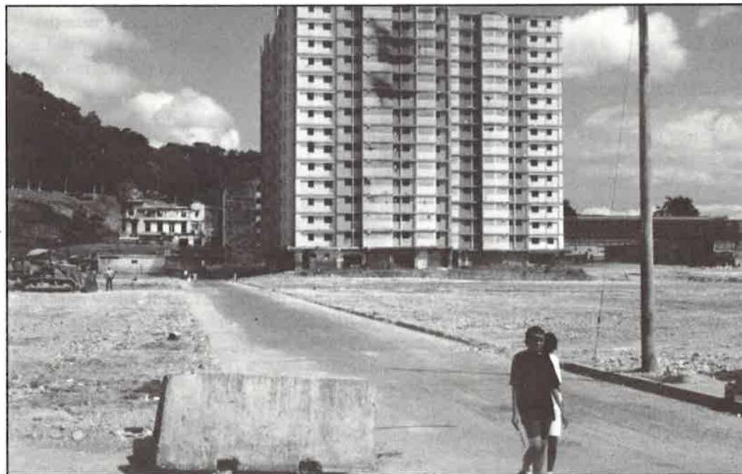
El Chorrillo after bulldozers cleared the wreckage.
