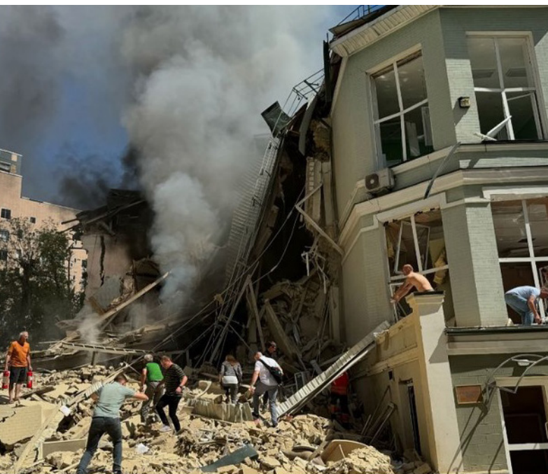
Image 5. The destroyed toxicology building at the Okhmatdyt hospital. Source: Okhmatdyt's Instagram 484
