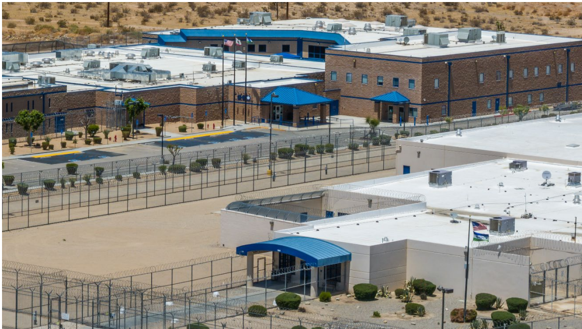
Immigration Customs Enforcement processing center which consists of East and West wings, located in Adelanto, California on May 18, 2025. © 2025 Getty Images
